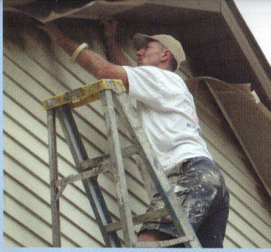
Terry Degue and his crew prefer Duration for aluminum siding and WoodScapes for cedar siding.
